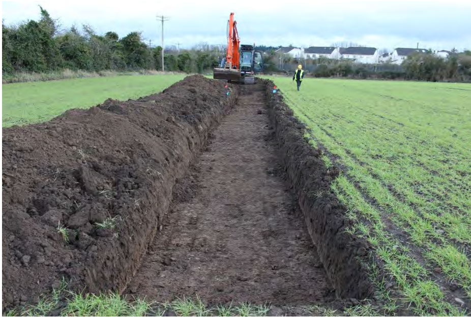
Plate 13: Trench 4a, looking south
