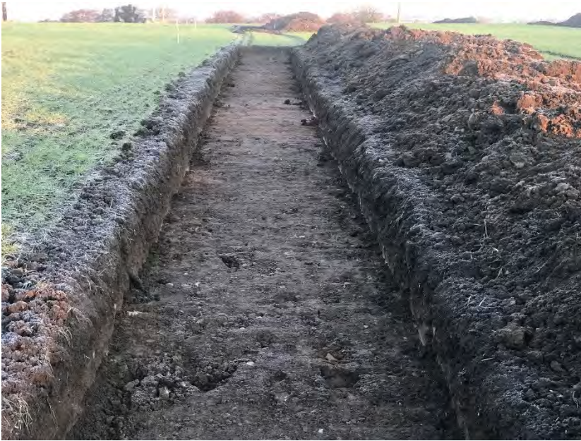
Plate 25: Trench 6a, variable in natural from stone to clay deposits
