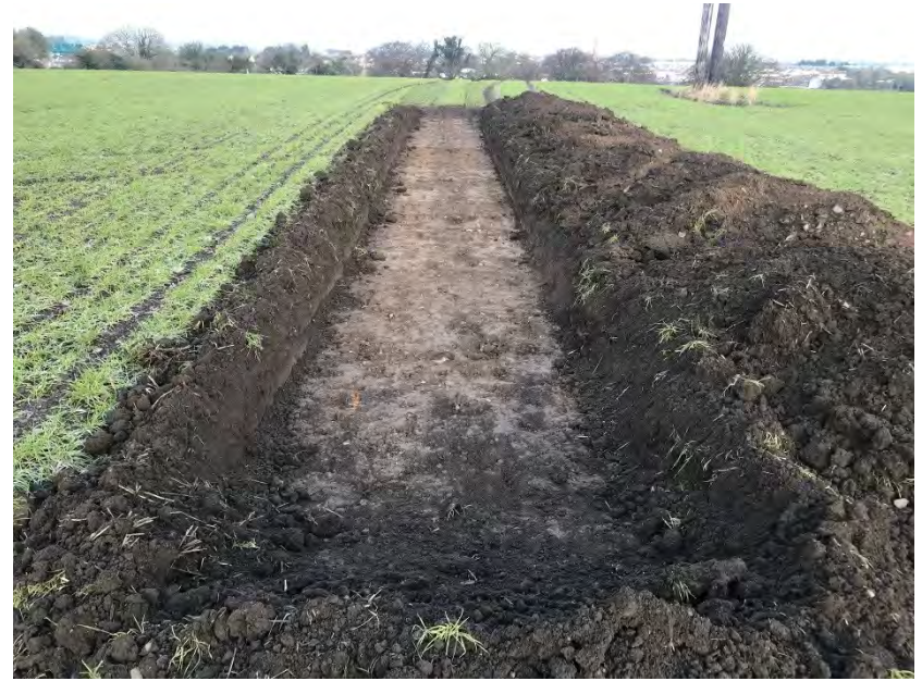
Plate 30: Trench 7b, looking north
