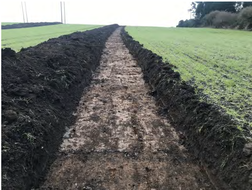
Plate 35: Trench 8c, looking south
