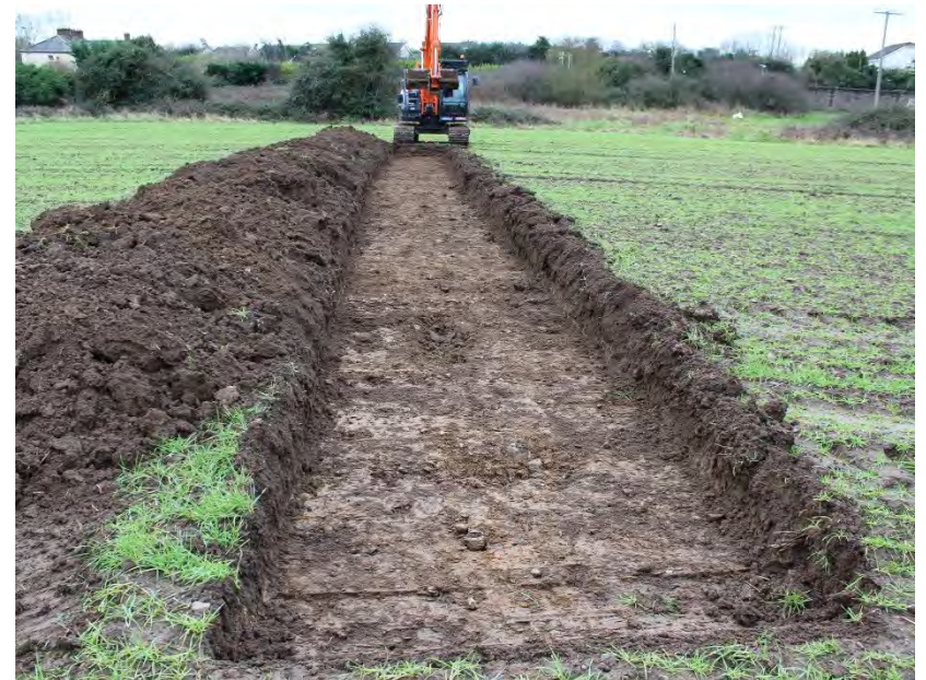
Plate 4: Trench 2a, looking south
